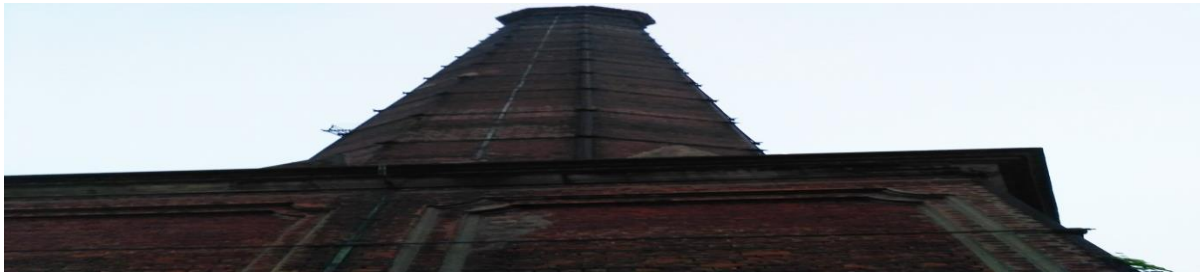
One of the defunct brick boilers of the Khardah Jute Co.
